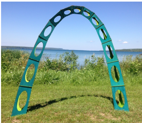
Figure 1: Catenary arch made of laser-cut wood pieces joined with cable ties. (6.5 feet tall)
