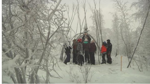
Figure 1: students constructing a qaluurvik, or willow frame house, in the western Canadian Arctic.
