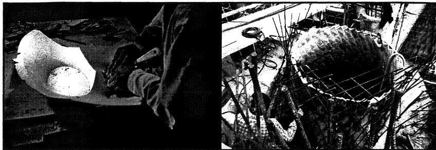
Figure 4-5: The plaster model of the nave window showing the straight line on the surface and the nave vaults under construction showing the application of the straight line geometry in the Catalan tile vaulting and in the placing of reinforcement
